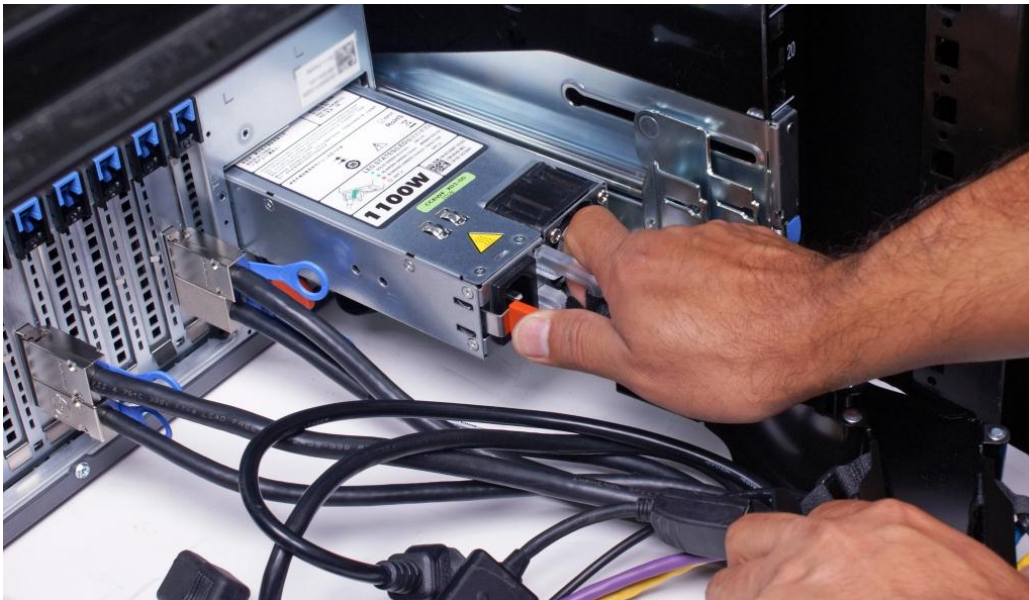
Figure 6. Replacing a hot swap power supply
